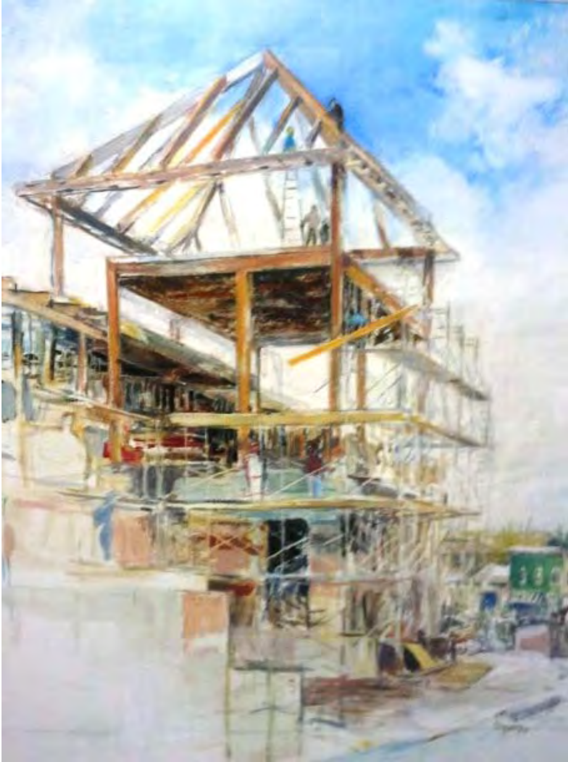
"A New Space: Saratoga Springs Public Library Under Construction" Anne Diggory, 1994
